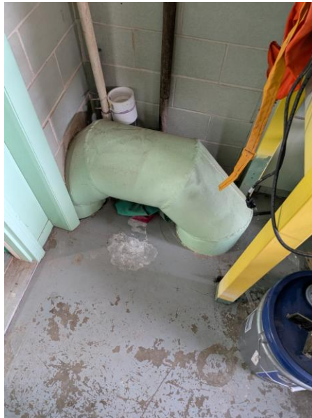
Transite pipe transitions to steel at this point on ground floor.
